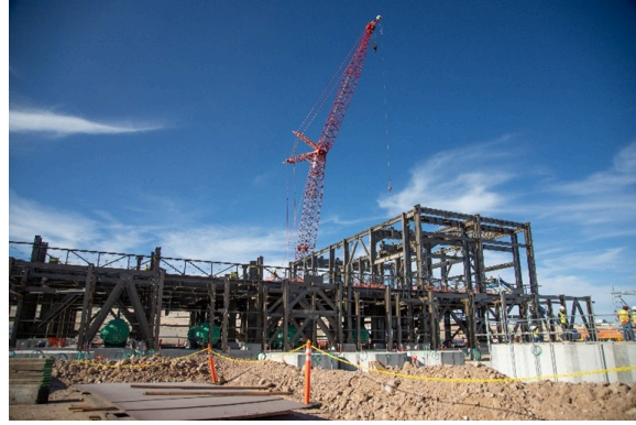
Figure D: Ring walls installed on one of eight counter-current decantation (CCD) units.
