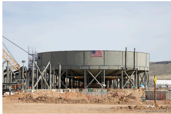
Figure D: Ring walls installed on one of eight counter-current decantation (CCD) units.
