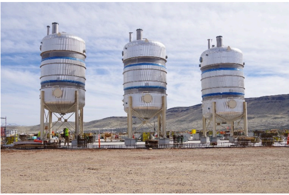
Figure C: Bicarbonate reactors for the Lithium Carbonate Crystallization facility have arrived at Thacker Pass.
