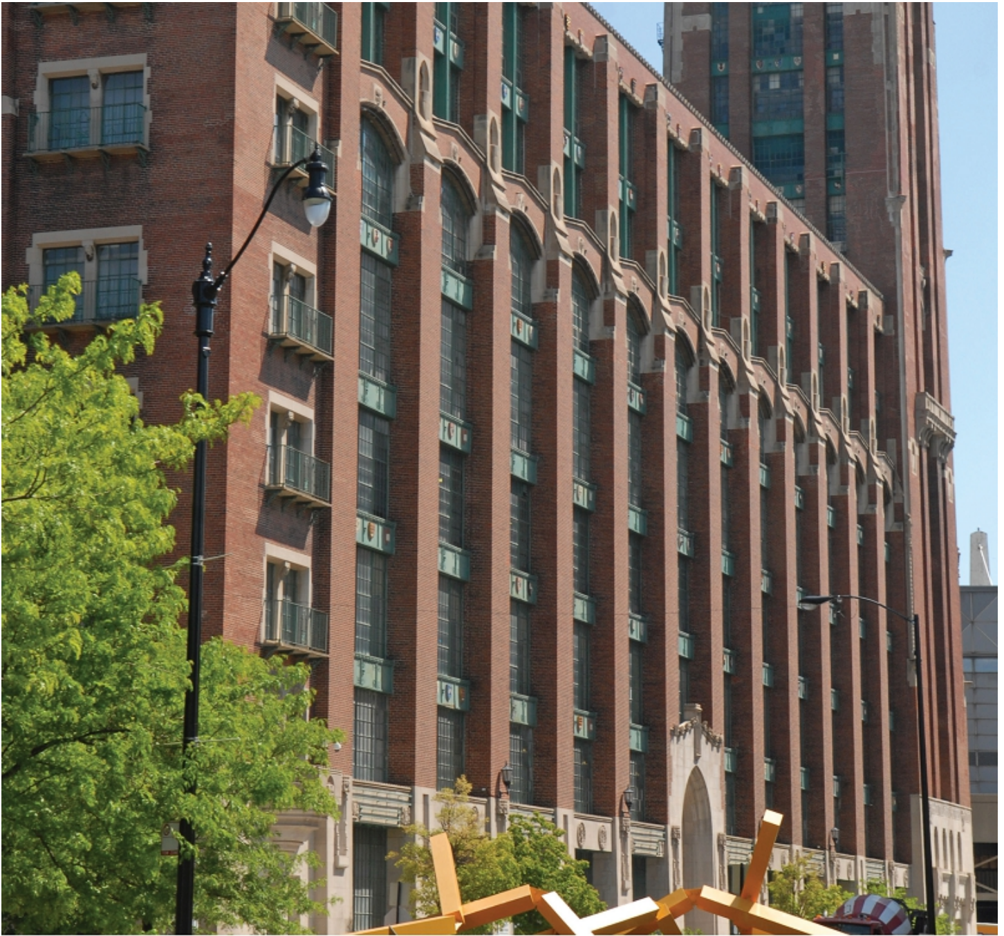
CH1, located in Chicago, Illinois, USA, is a former printing facility.
