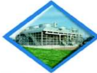
Recovered Energy Power Plants Enterprise, Louisiana
