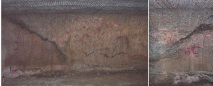
Figure 6-6: Wash-out Anomaly
