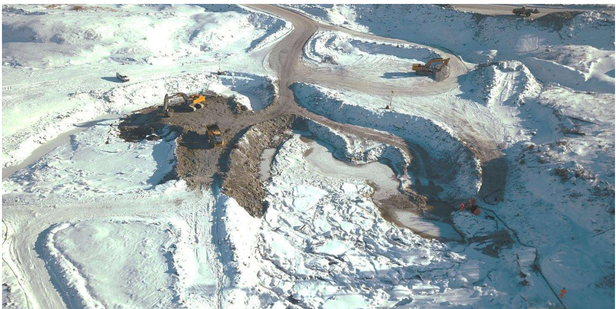
Côté Gold – TMF Starter Dam Foundation Excavation (January 2022)
