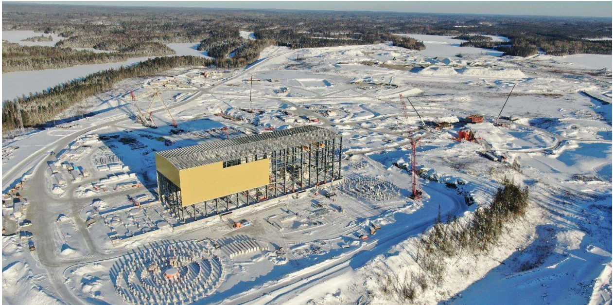
Côté Gold – Processing Plant Wall Panel Cladding (January 2022)
