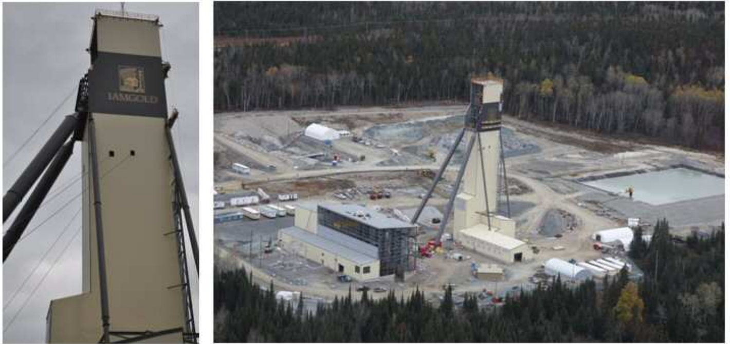
Figure 1 : Westwood Development Project, December 2009
