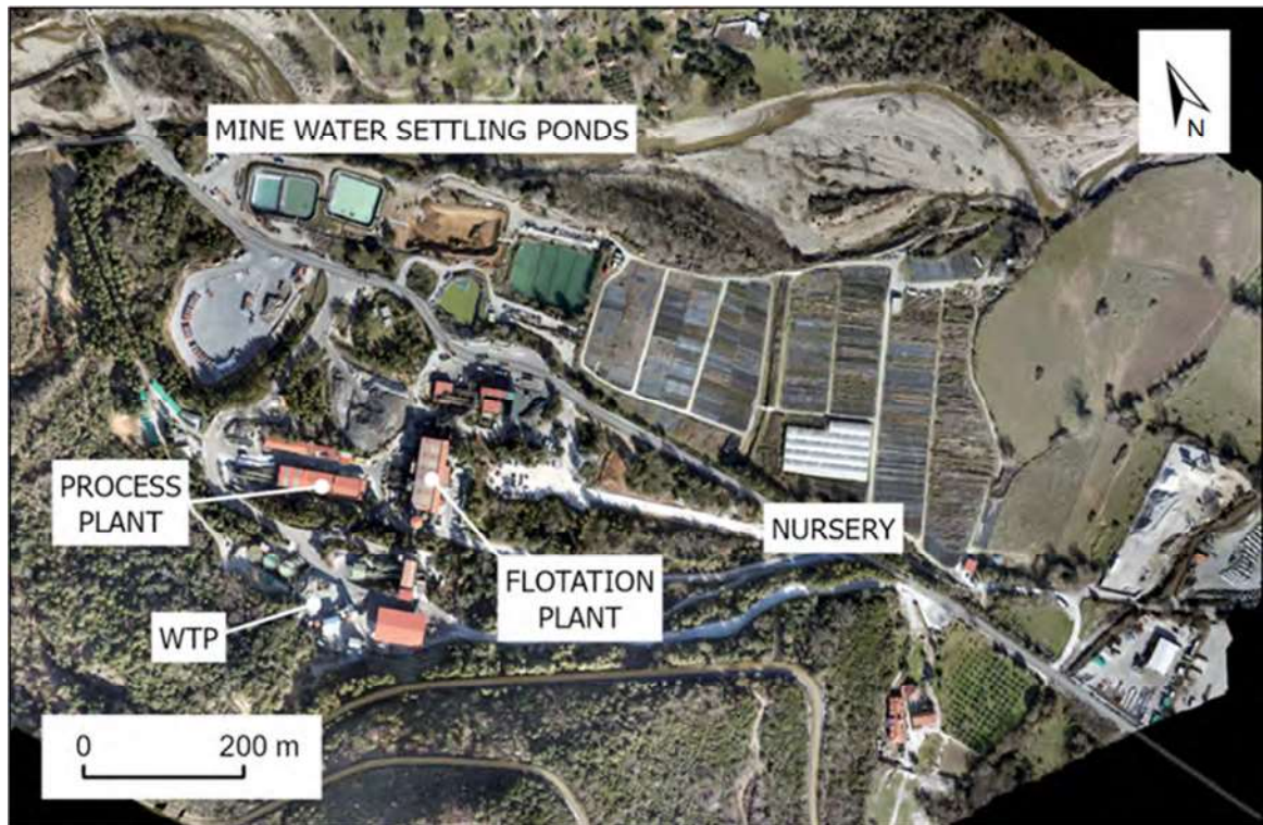
Figure 18-3: Olympias Process Plant (Eldorado, 2023)
