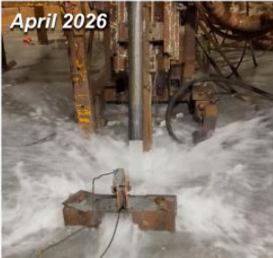
Two drill holes making water
