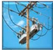
Supervisory Controlled Switches
