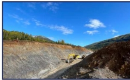
Pond 5 tailings project
