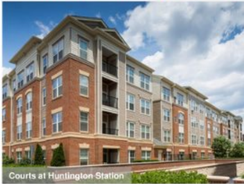
Courts at Huntington Station
