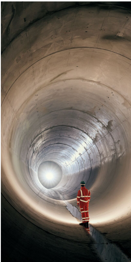
Leveraging our experience in delivering critical infrastructure programs end-to-end, we've been the program manager for the Thames Tideway Tunnel since 2008. Now operational, the new super sewer will dramatically reduce sewage pollution, creating a cleaner, healthier River Thames and a positive legacy for London, U.K.
