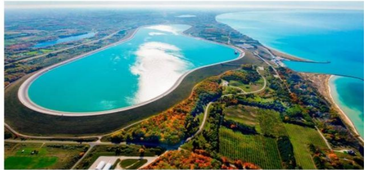
Ludington Hydropower Plant
